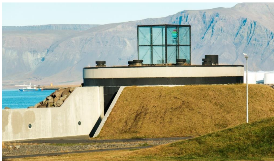
Figure 4: Sewage treatment plant at Eidisgrandi in Reykjavik City. Photo: Einar Örn Jónsson
